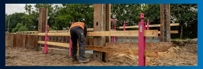
Both crossbars fully inserted. The height to the top edge of the upper transom is approx. 1150 mm.
