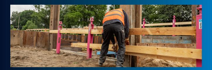
Insert the spars by hand. Initially, work in front of the shoring and later always next to the already installed tie-bars. The worker is therefore always in the secured area.
